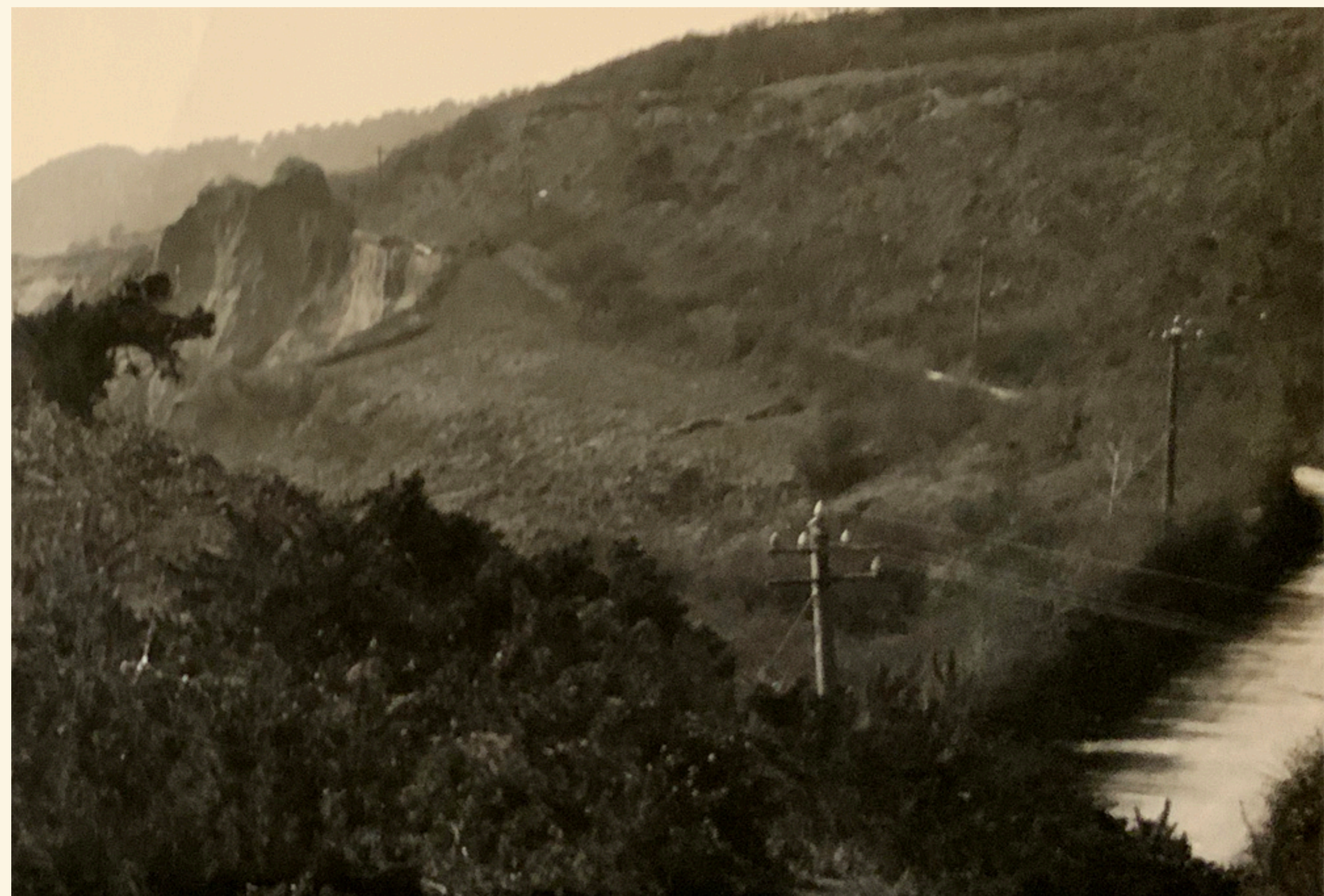
Close up of road before landslide
