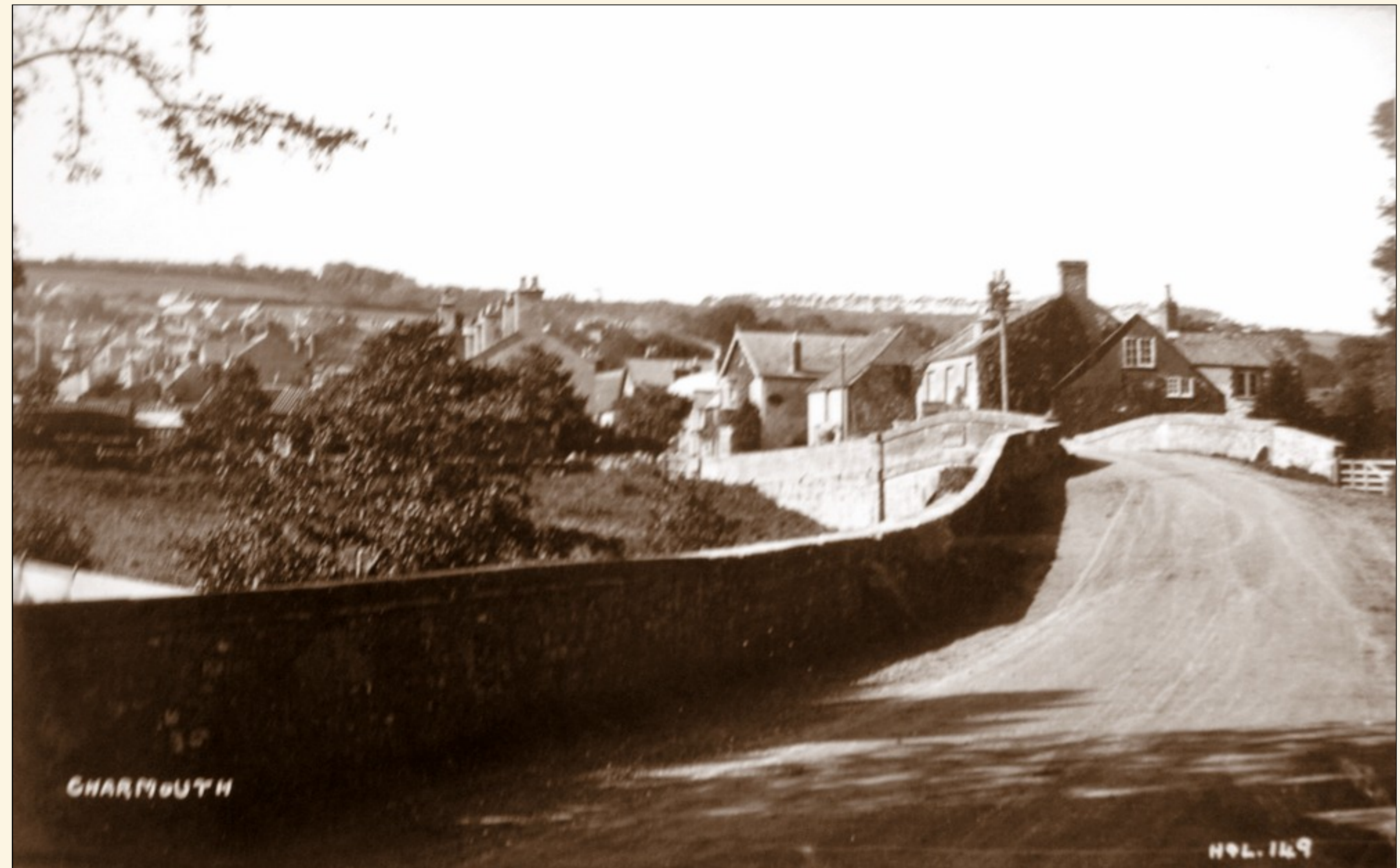
A real photo postcard of the County Bridge as it enters The Street in Charmouth by H&L ( Hider & Lawrence)
