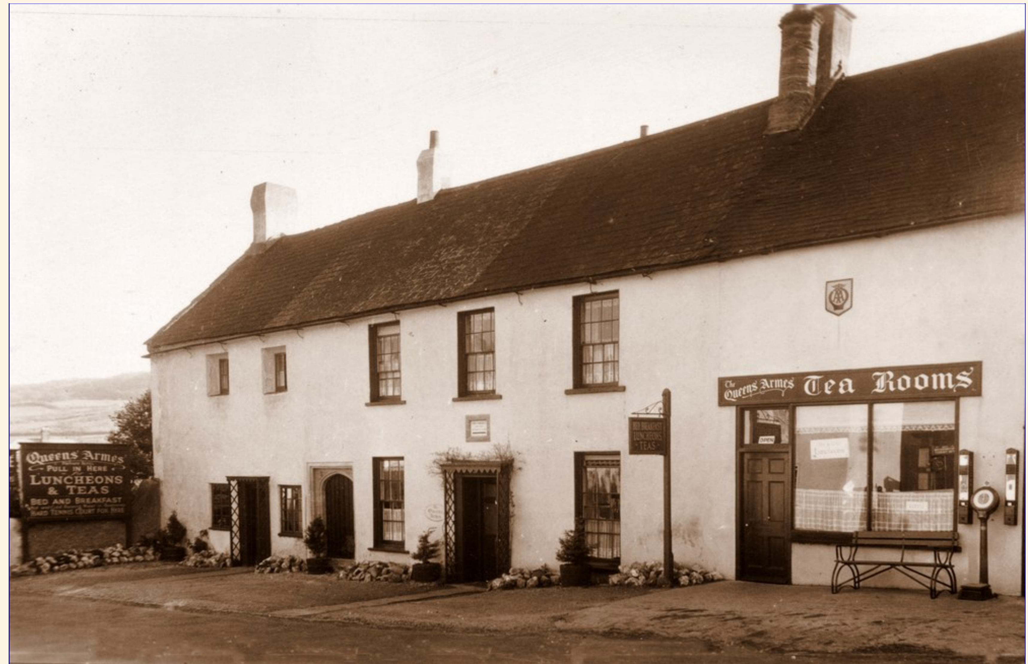
Claude Hider often returned to take updated photographs, here he shows the former Manse as a hotel and Tea Rooms after restoration . The building is now Known as "The Abbots House" which relates to its links with Forde Abbey.
